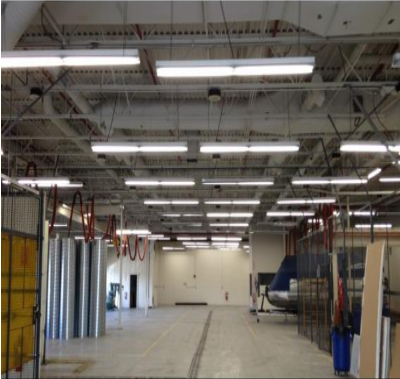
High Bay Space Interior: 21' Clear
